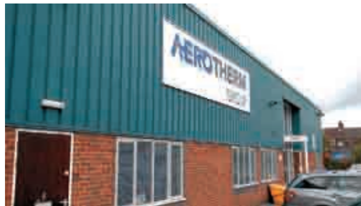
COUNCIL SUPPORT... Aerotherm's new, bigger premises at Scotia Business Park, Tunstall have helped the company stay in the city and create jobs.
